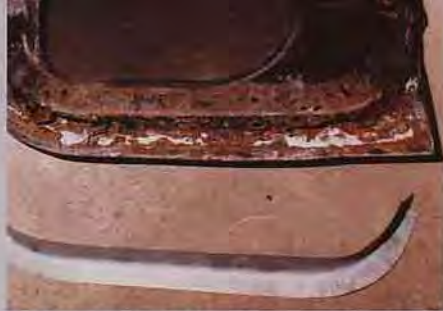
The door bottoms can rot out badly. Photo:- Dennis Doubtfire.
