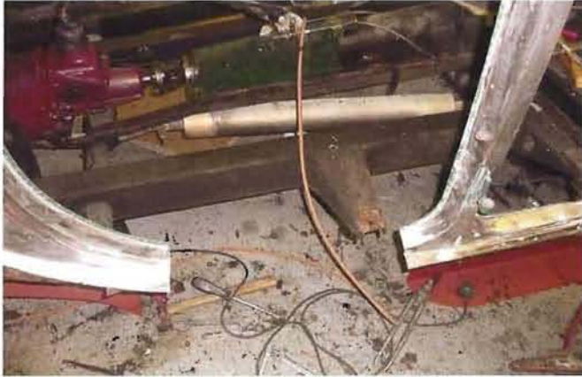
The dodgy metal has been cut out ready for the repair panel.
