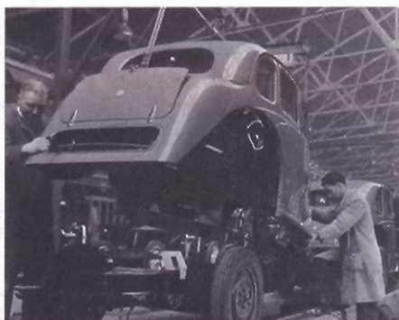
The trimmed body shell is lowered from the top deck to be united with its rolling chassis. From then until it moves under its own power the car remains on the one production line
