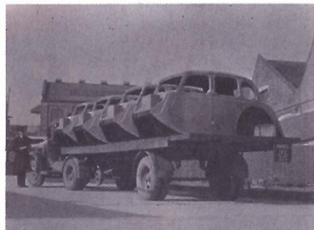
Painted bodies were delivered from Cowley to Abingdon where they were delivered to the top deck of the factory for trimming
