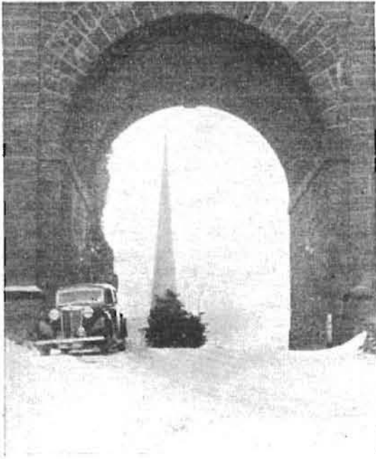
TOPSY-TURVY. —To emerge from a tunnel and suddenly look down upon the church spires is typical of precipitous Luxembourg.
