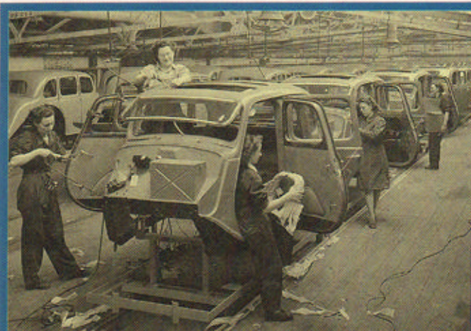
On the "top deck", women workers (above left) installed all the trim and many minor components before the bodies were fitted to the chassis. Above right: Nearing completion, with seats installed and wings fitted, only a few tasks remain to be carried out.
