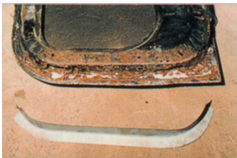
2. ... for although the doors looked in excellent nick, they were little more than rust with filler. Steve ended up fabricating his own repair sections.
